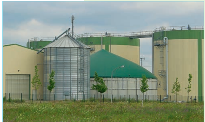
Flexible plant design is adaptable to site requirements
